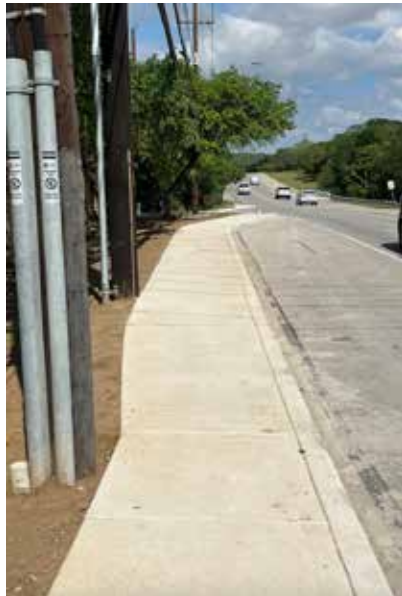
Looking north on Lockhill-Selma to the end of the project.
