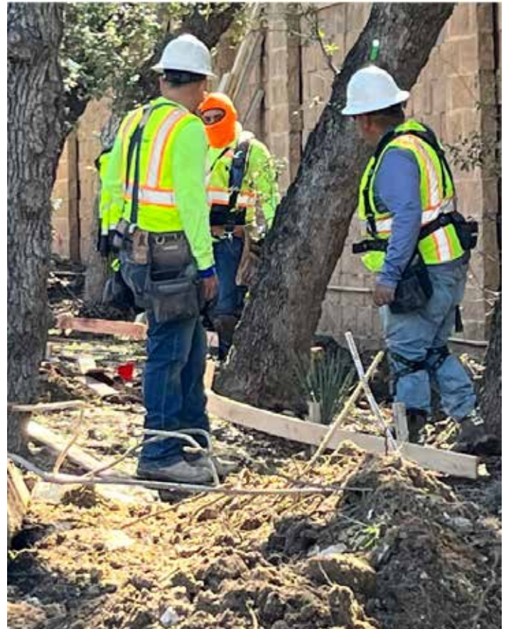
Workers set sidewalk guides to avoid cutting down a tree.
